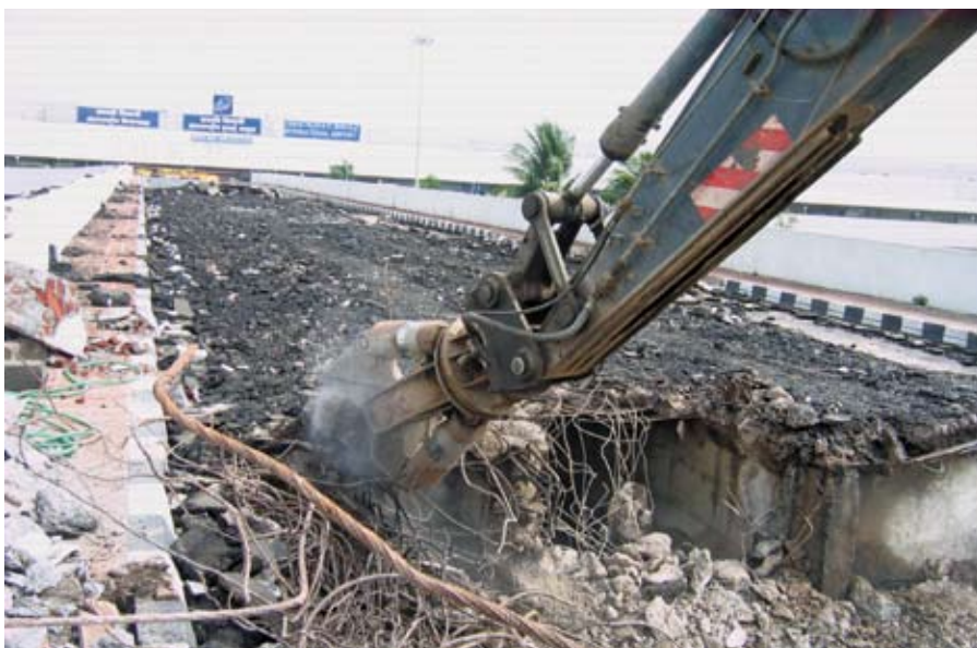
Demolition of ramp at Mumbai International Airport Ltd.
