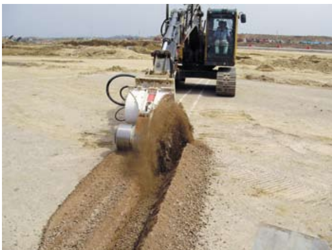
Concrete trenching using Drum cutter at Delhi International Airport, New Delhi
